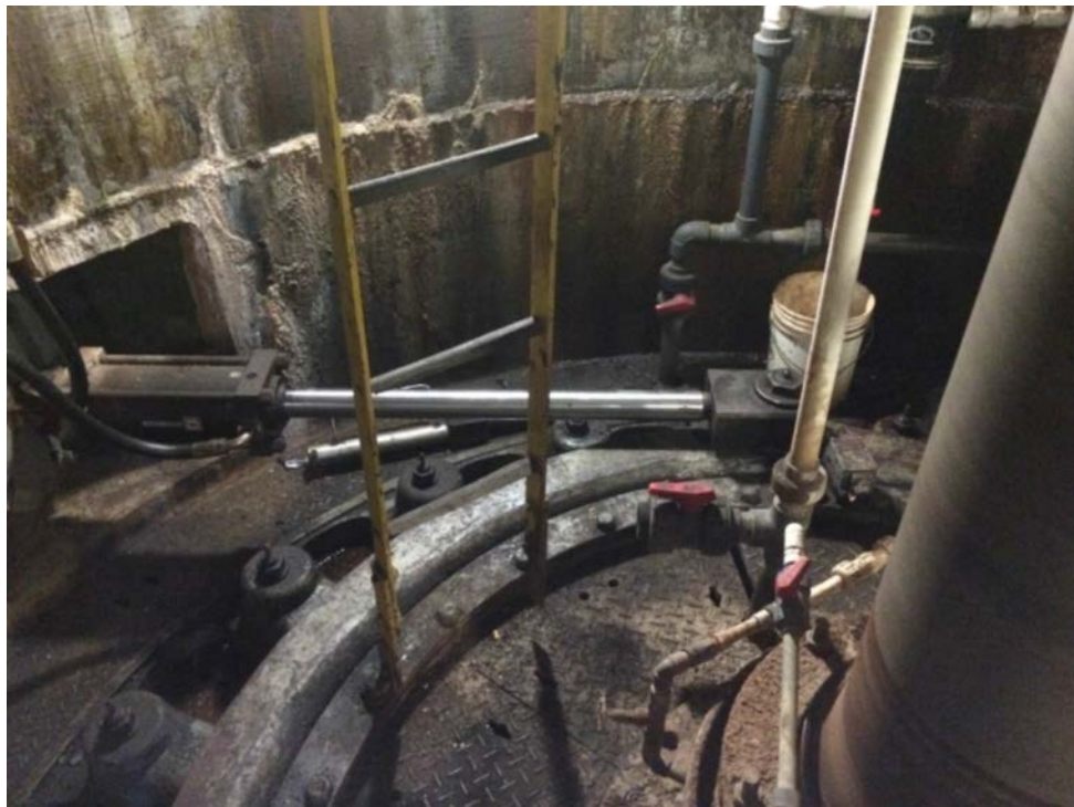
PHOTO 4-1 PARR SHOALS DAM PIPING FOR VACUUM BREAKERS IN HEADCOVER
